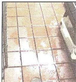
Watch for liquid on the floor. Clean up spills. Report conditions.
