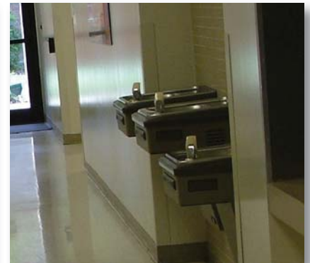
Water fountain area.
